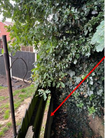
Trunk and root plate slowly pushing concrete fence out of line and into the neighbouring garden.
